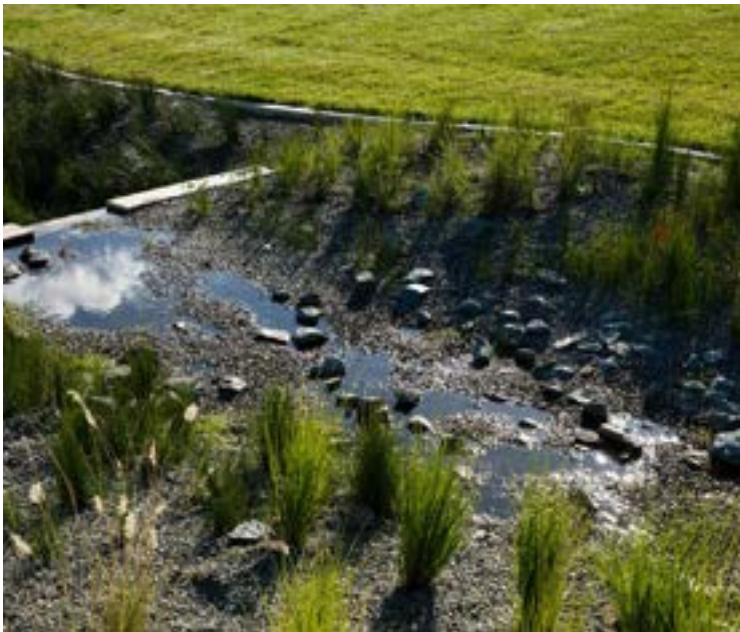
3.4: Passive irrigation and rain gardens.
