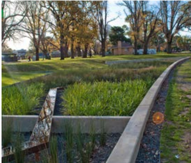
3.2: An example of a raingarden that will be located within Reaburn reserve to clean stormwater.
