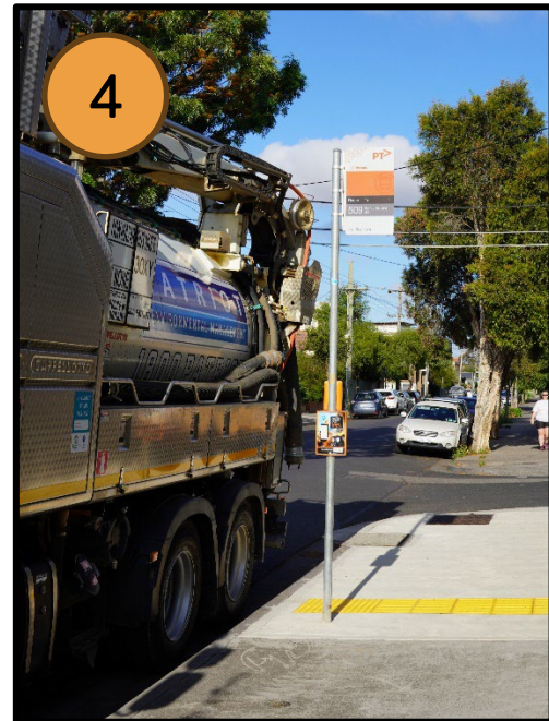
Bus stop with tactiles
