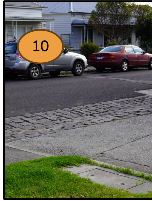
Concrete Road intersection at Ferry Street
