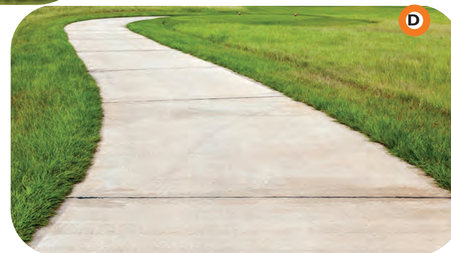
New concrete path connecting to seating and court through existing low brick wall opening
