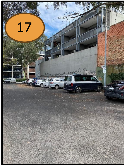
Car Park behind 36 Breese Street
