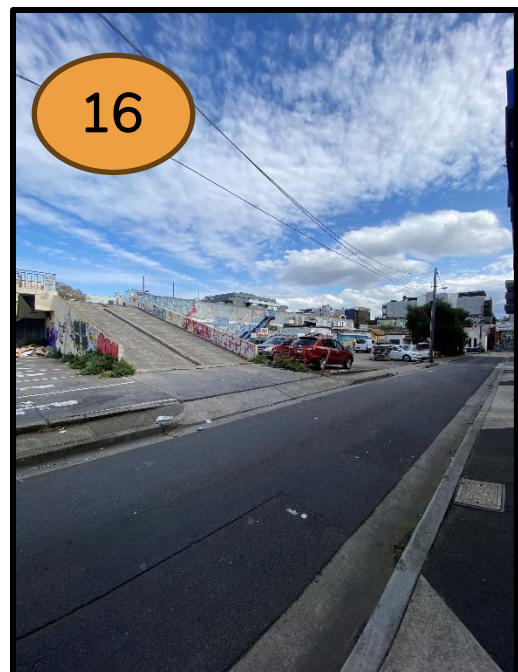
William Street Private Car Park
