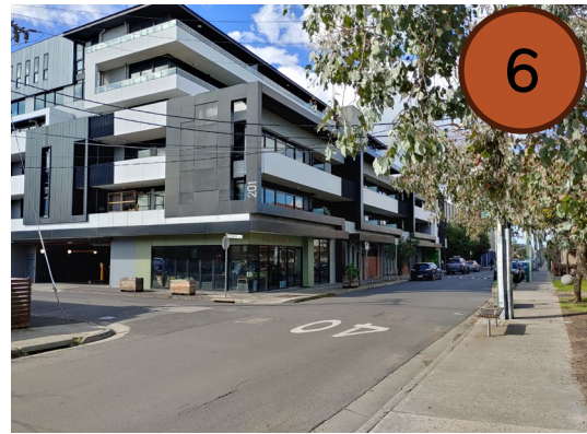
Albert Street at Randazzo Park looking east
